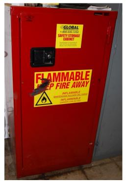
Flammable storage cabinets are required for flammable materials. These come in many different sizes depending on the amount of material to be stored. A maximum of 60 gallons of category 1,2, or 3 liquids can be stored in a single cabinet and no more than 3 cabinets are allowed in a storage area.
