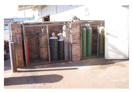
Gas storage – Cylinders should be clearly marked. Oxygen must be separated from fuel.
