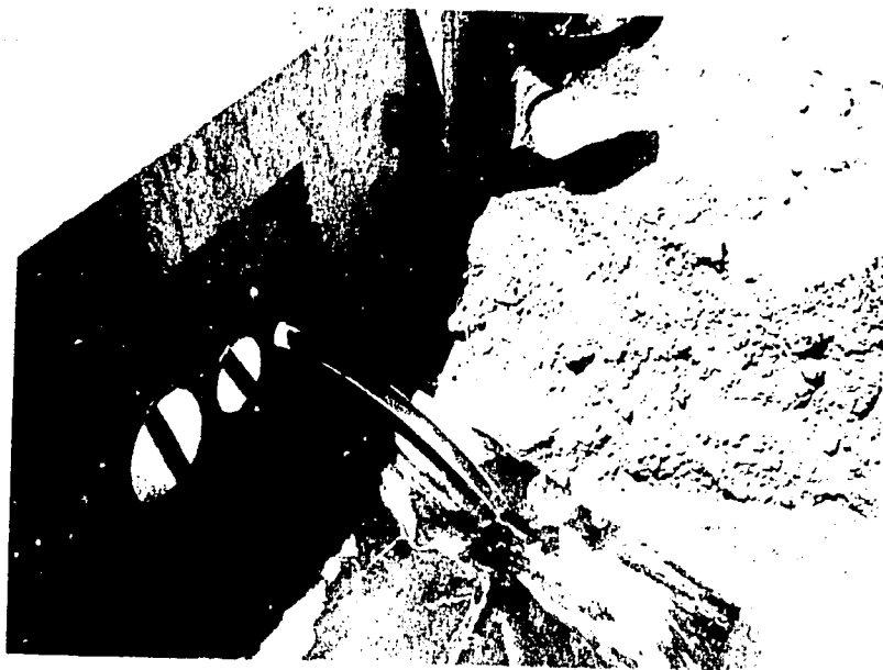
Figure B-2. Orifice board installed for a furrow test with only one orifice open.
