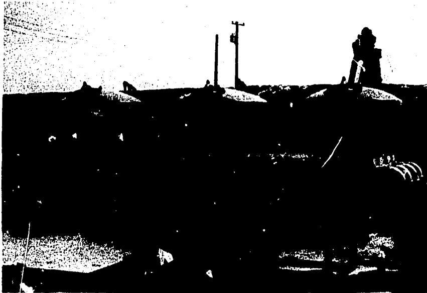
Figure VIII-3. Typical bank of sand filters followed by screen filters for a trickle irrigation system.
